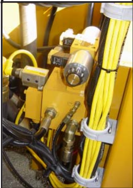
Figure 7-D. Clamp Manifold Installed
